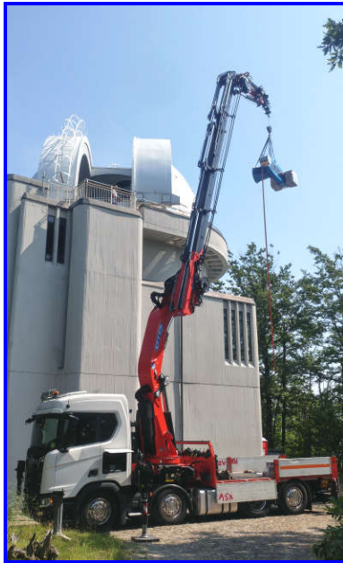
Figure 8 – Two views of the TANDEM final installation at the Loiano Observatory, on June 27, 2023. Left panel: TANDEM on its way to the Cassini dome, dangling from the crane. Right: inside the dome and close to its final anchoring to Cassini.
