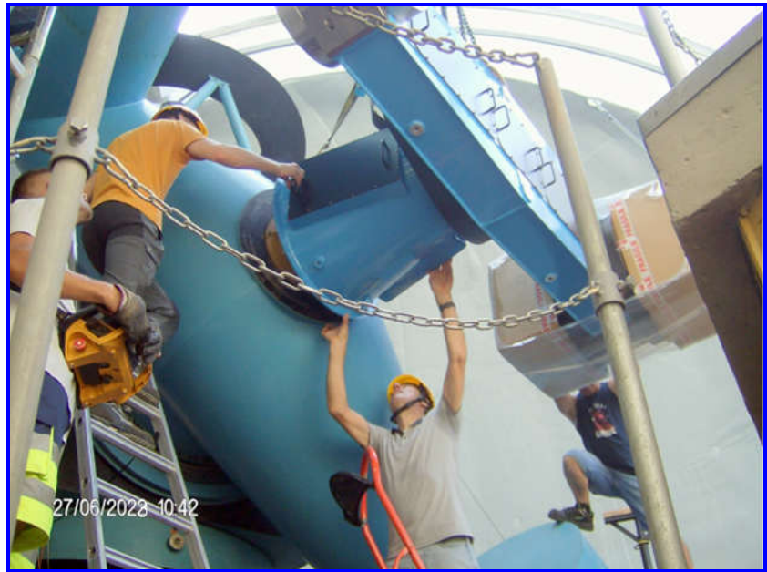
Figure 8 – Two views of the TANDEM final installation at the Loiano Observatory, on June 27, 2023. Left panel: TANDEM on its way to the Cassini dome, dangling from the crane. Right: inside the dome and close to its final anchoring to Cassini.
